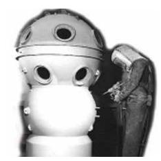
Zinc metal sprayed coatings being applied to the outer and inner surfaces of a Diving Bell.
