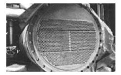
This Condenser End Plate was fully rebuilt with Ceramic Metal using specialised application techniques.
